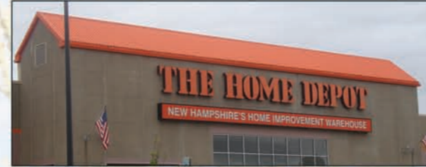
Cement Block Construction
